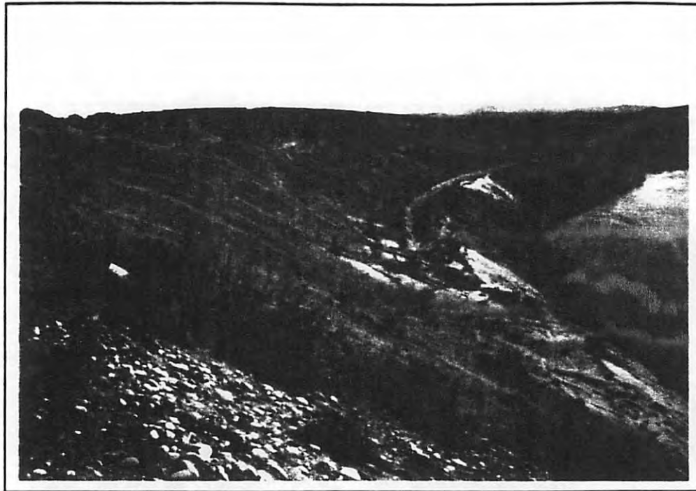
Figure 2. View to east from west of escarpment. Off-road vehicle tracks have denuded areas uphill of the the can, precipitating erosion. Note that abandoned canal is filled with eroded soil from uphill.
